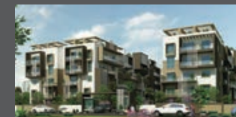
VRR STONE ARCH, OFF HENNUR MAIN ROAD
